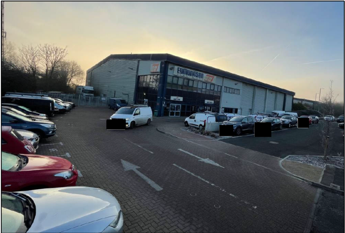
Plate 3: Image of EEL Access and Area Covered by DCO Application Order Limits
